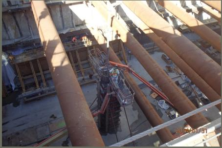
Column and Wall formwork in progress
