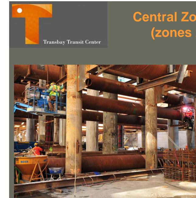
Bracing removal continues in preparation for wall and Lower Concourse formwork
