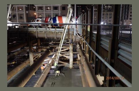
Completion of 80% of the central zone lower concourse level slab has allowed for the placement of 3<sup>rd</sup> lift foundation walls and re-bracing. These are the items that need to be completed prior to start of structural steel.
