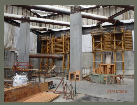
Completion of perimeter lift 2 walls and internal concrete walls prior to start of Lower Concourse decking.
