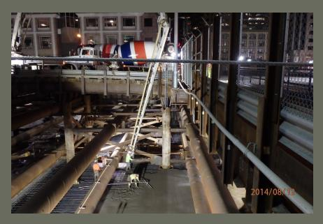
Completion of 80% of the central zone lower concourse level slab has allowed for the placement of 3<sup>rd</sup> lift foundation walls and re-bracing. These are the items that need to be completed prior to start of structural steel.
