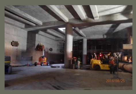
Rail Level in central zone is clear of internal bracing.
