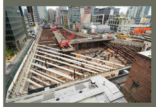
Primary focus in the western zone has been the completion of the Lower Concourse level decking for concrete placement.
