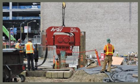
Installation of shoring at Pylon 9 location in preparation for Barrette Pile installation work has been completed. Cable-stayed pylon structure requires the specialized barrette pile foundation to accommodate lateral seismic forces without impacting train box.
