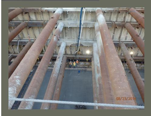
Mat foundation slab placement #15, reinforcing steel for mat foundation pour #16 (the last one).
