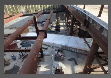
Above Left: West end train platform level with lower concourse formwork removed.
