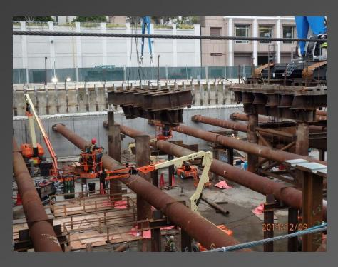
Above and Right: Removal of next section of access trestle for continuation of steel erection.
