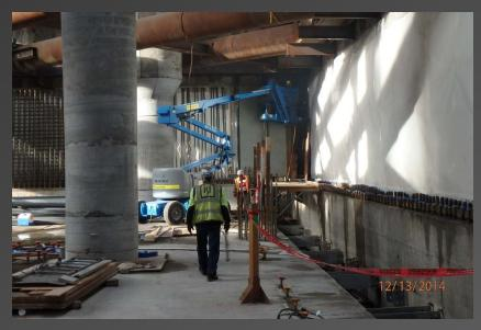
Above: East wall first lift, waterproofing in place.
