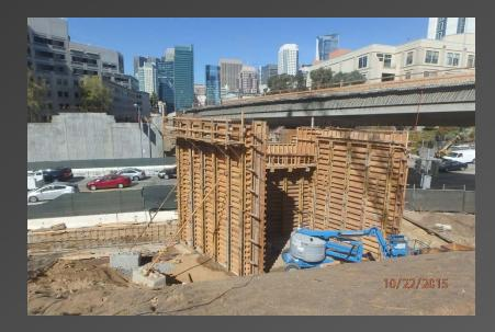
Above: Abutments and retaining walls at Harrison Street. Above Right: Viaduct formwork and reinforcing steel at Frame 1. Below Right: Viaduct formwork, reinforcing and embedded items in Frame 3.
