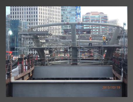
Above: Light column welding now complete. Above Right: Trainbox lid "eyebrow" formwork at south side. Below Right: Preparing light column base plate bolts.
