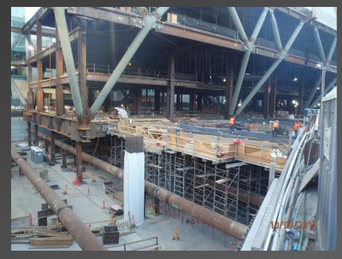
Above: Formwork for trainbox lid at southwest corner. Above Right: Trainbox lid "eyebrow" formwork at north side Shaw Alley. Below Right: West and central zone structural steel is now connected.
