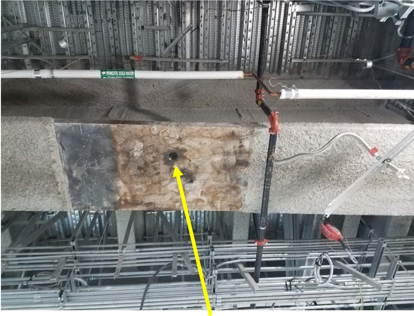
Core sample taken to advance testing process
