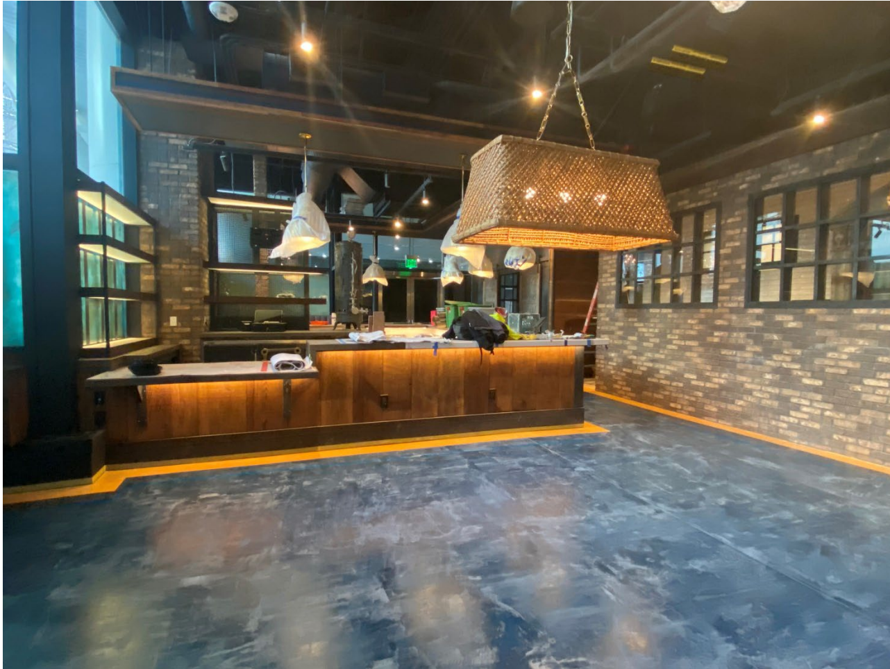
Per Diem; Flooring completed
