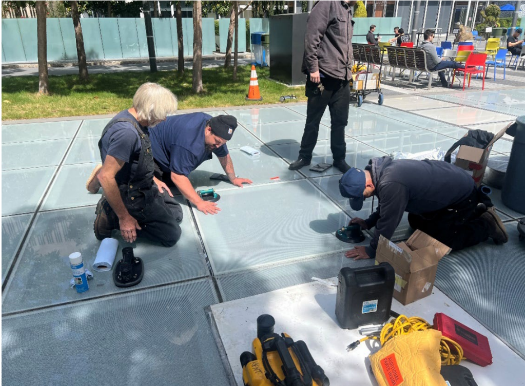
Salesforce Park, glass replacement in the Main Plaza
