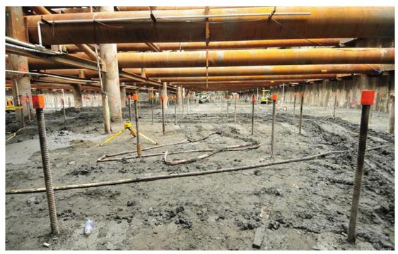
Rows of orange-tipped micropiles line the lower level of the Transit Center "Train Box"
